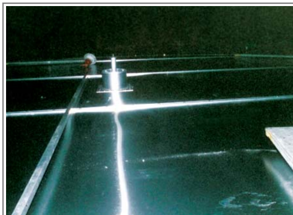
Pressure & Vacuum Breaker System
