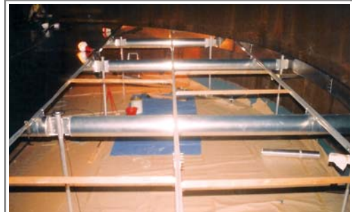
Inside View of WBIFR Assembling Work in Japanese Oil Company, 1999 March
