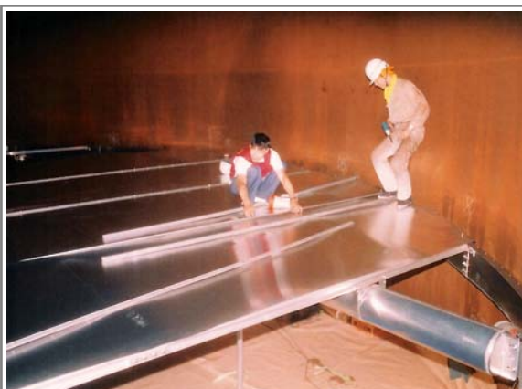
Deck Skin Assembling Work / Japanese Oil Company
