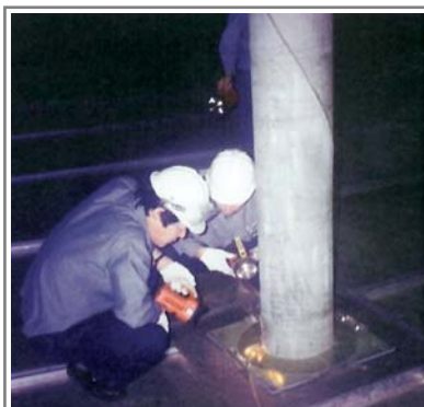
WBIFR Column Well Inspection Work in Local SK Corp. Oil Storage Tank
